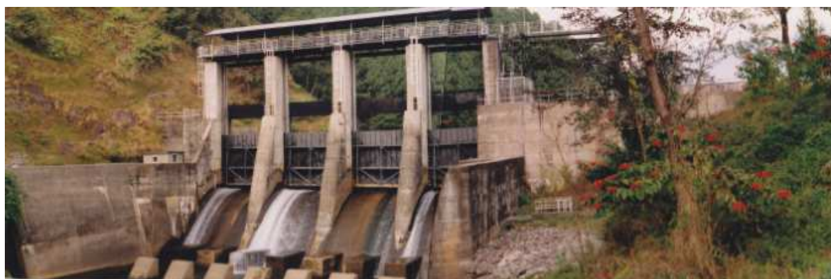
DamSite,Fewa Lake Hydro Plant
