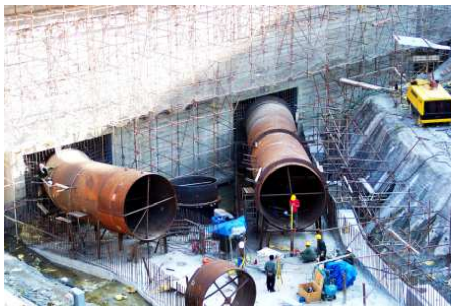
Penstock Construction, Mid Marsyangdi Hydro Power Plant
