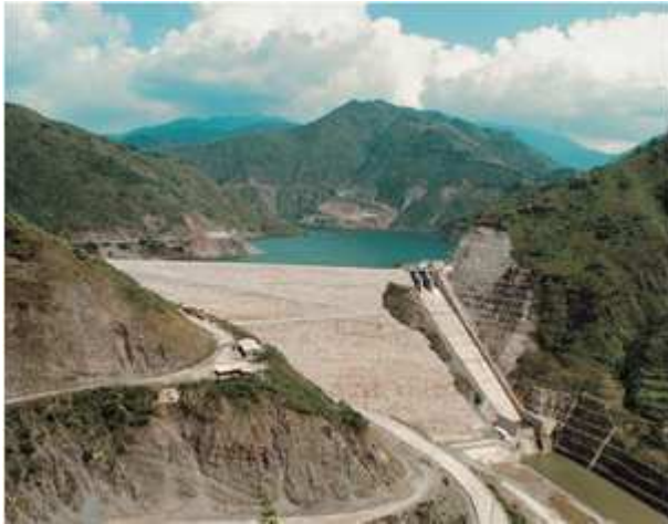
Kulekhani-1, Dam site.
