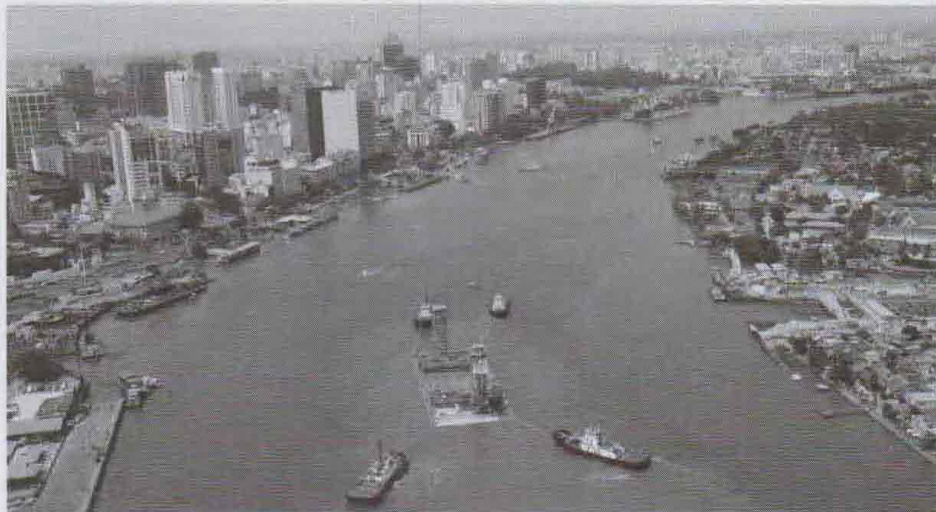
Towing of Immersed Tunnel Unit 1 for immersion in Saigon River, March 2010
