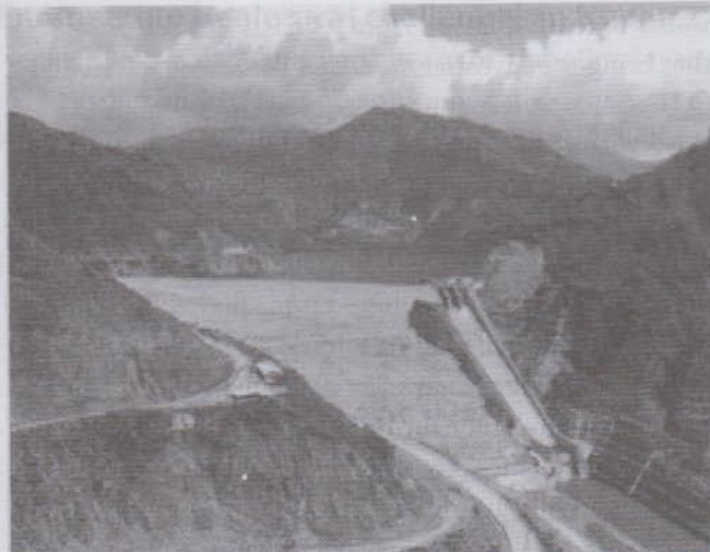
Kulekhani-1, Dam site
