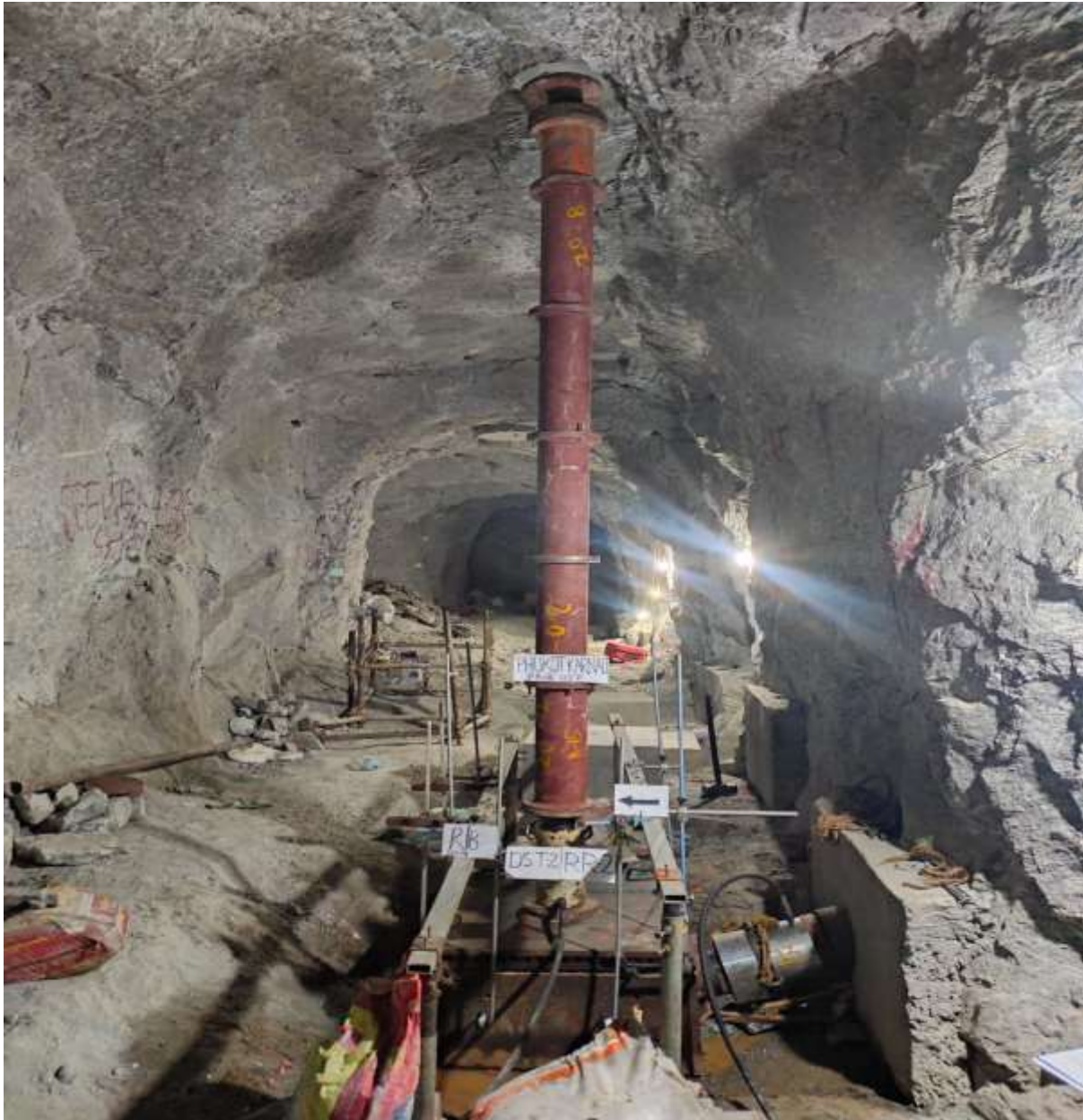
Fig.16- shows the in-situ-Load Test in Tunnel.
