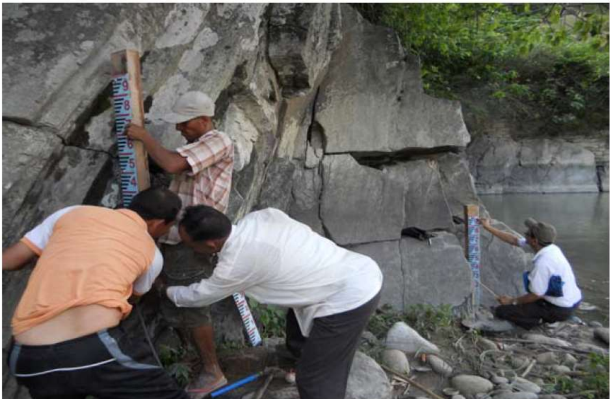
Fig.5- Installation of Staff Gauge on the riverbank.
