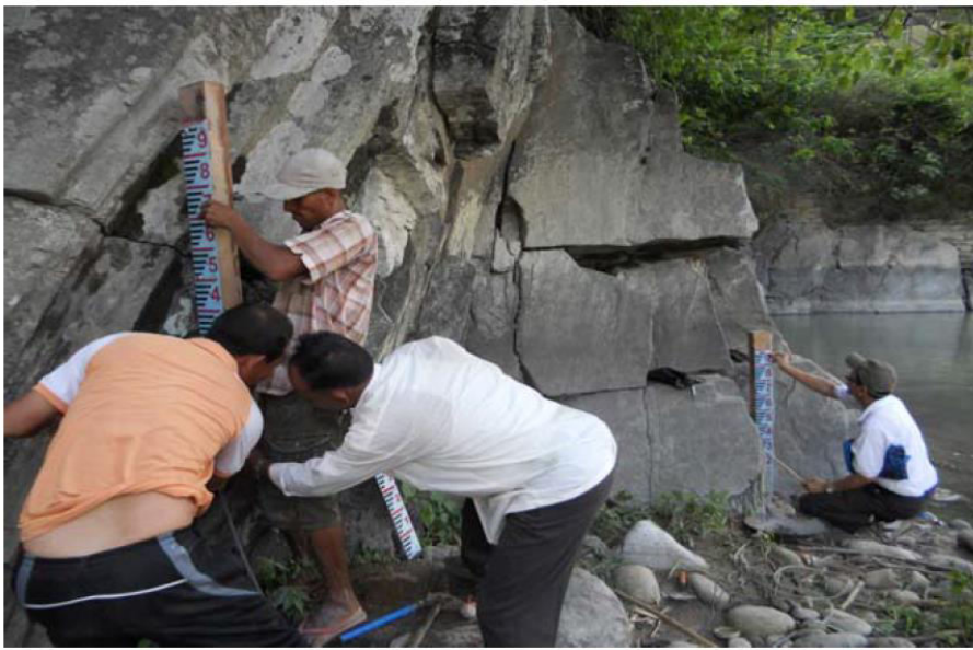
Fig.5- Installation of Staff Gauge on the riverbank.
