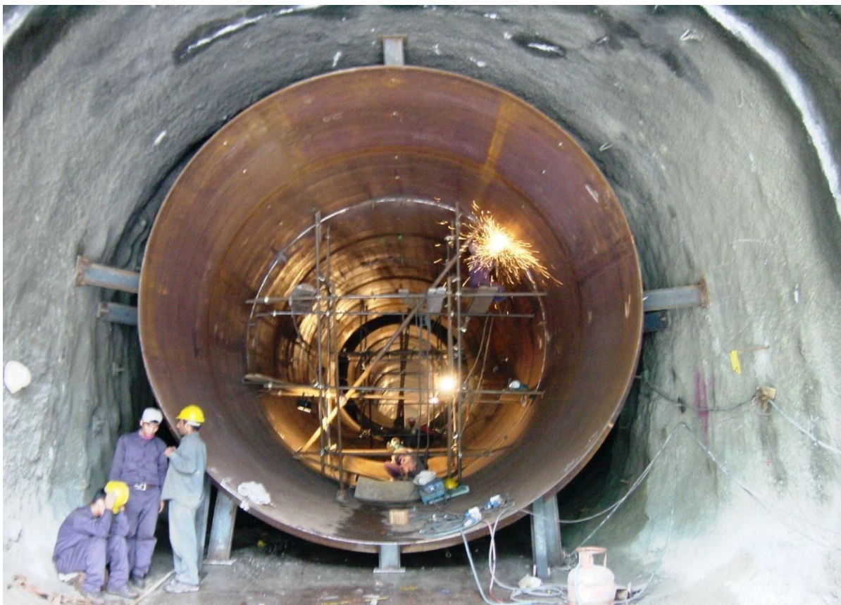
Fig.5 Welding of steel liner in the penstock tunnel(Typical)
