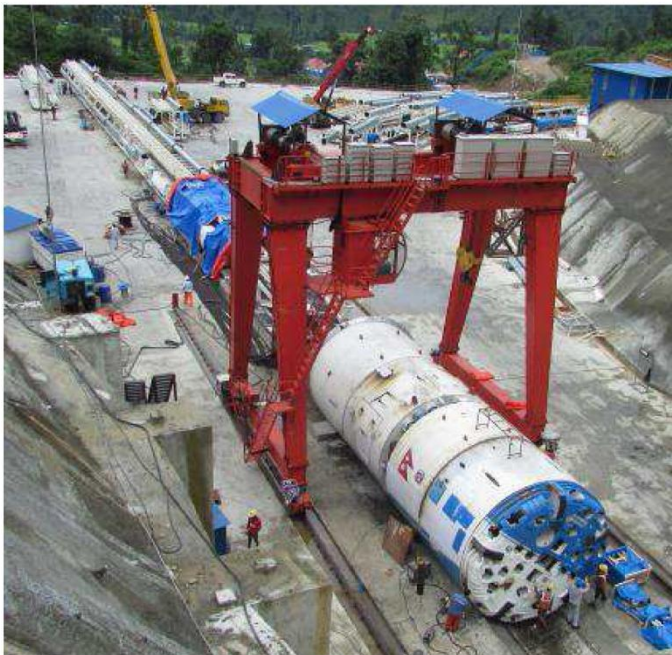
Fig 9.1 Showing the TBM in Bheri Babai Project
