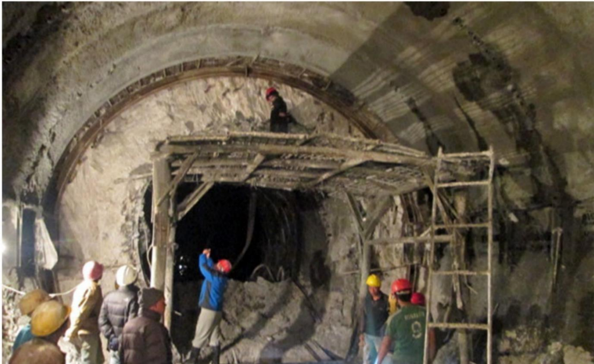
Fig.1. Treatment of Tunnel Squeezing in the Chameliya HEP
