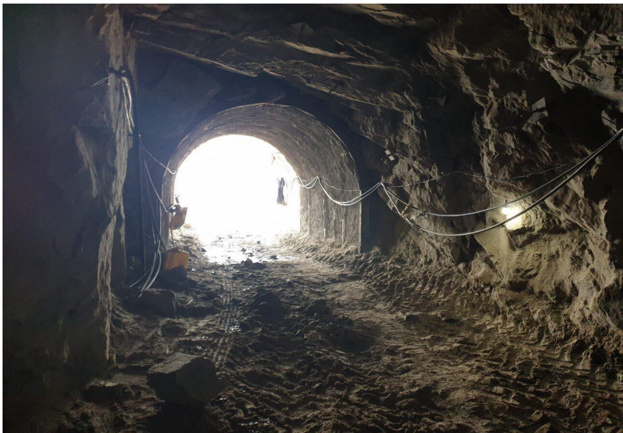
Fig.2 Tunnel Portal under construction.
