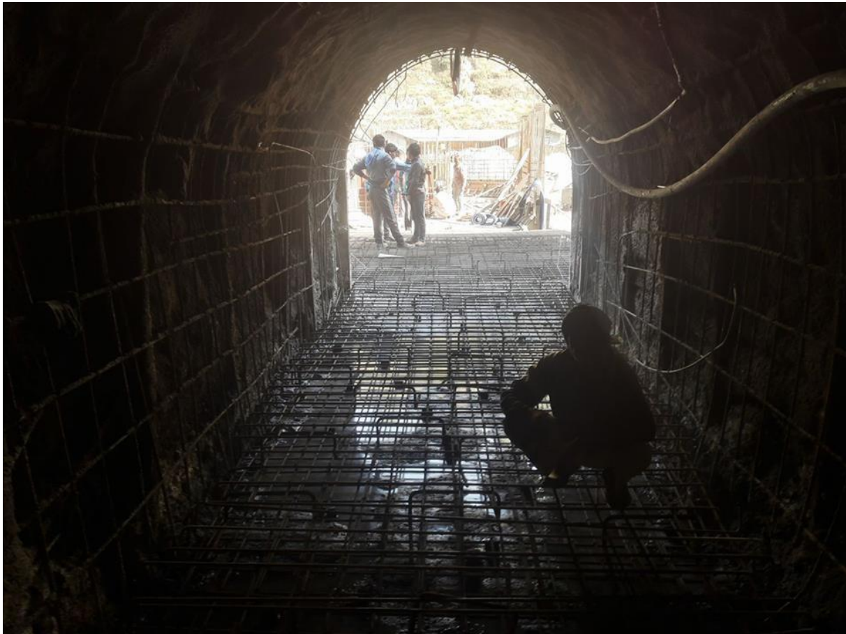
Fig.4 The reinforcement work in the RCC Lining of Tunnel (Typical)
